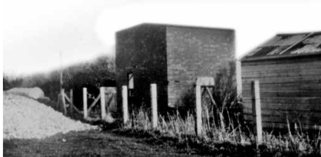
Seaton brick-built above-ground post at the Seaton Down Hill site. Note the post hut on the right. The pile of debris on left might be the material from the nuclear post excavation which could date the photo to c1959
